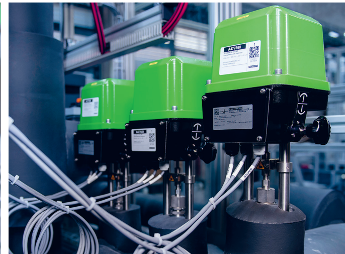
The precise sliding gate flange motor valve 8038 from Schubert & Salzer meets the demanding requirements.
