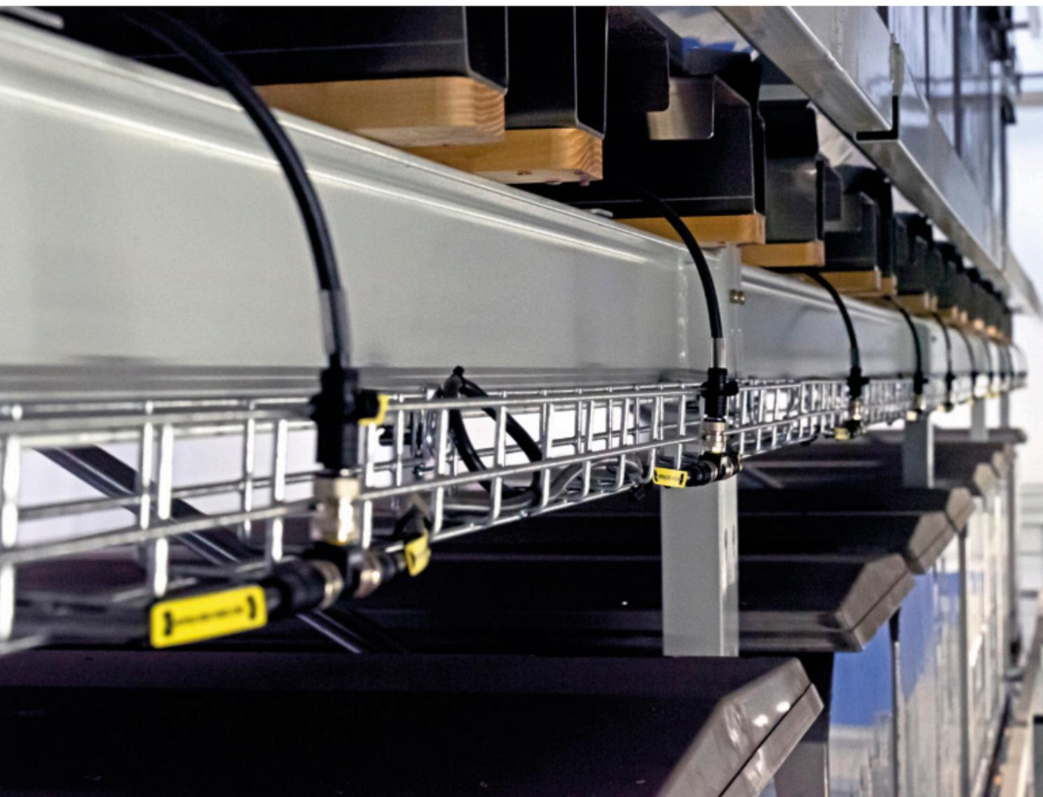
Thanks to Turck's HF bus mode, the HF read/write device can be connected very easily to each shelf rack using T pieces, thus considerably reducing wiring effort and costs
