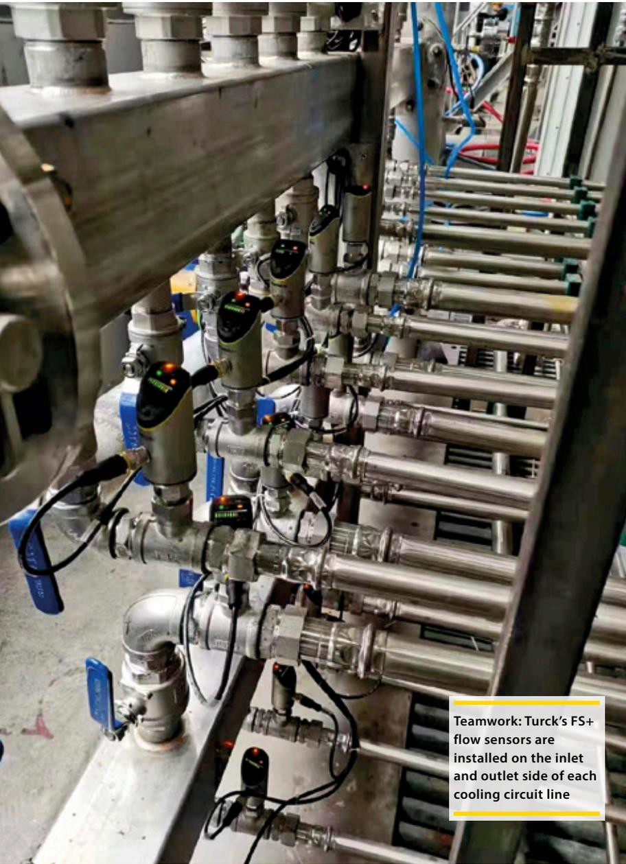
Teamwork: Turck's FS+ flow sensors are installed on the inlet and outlet side of each cooling circuit line
