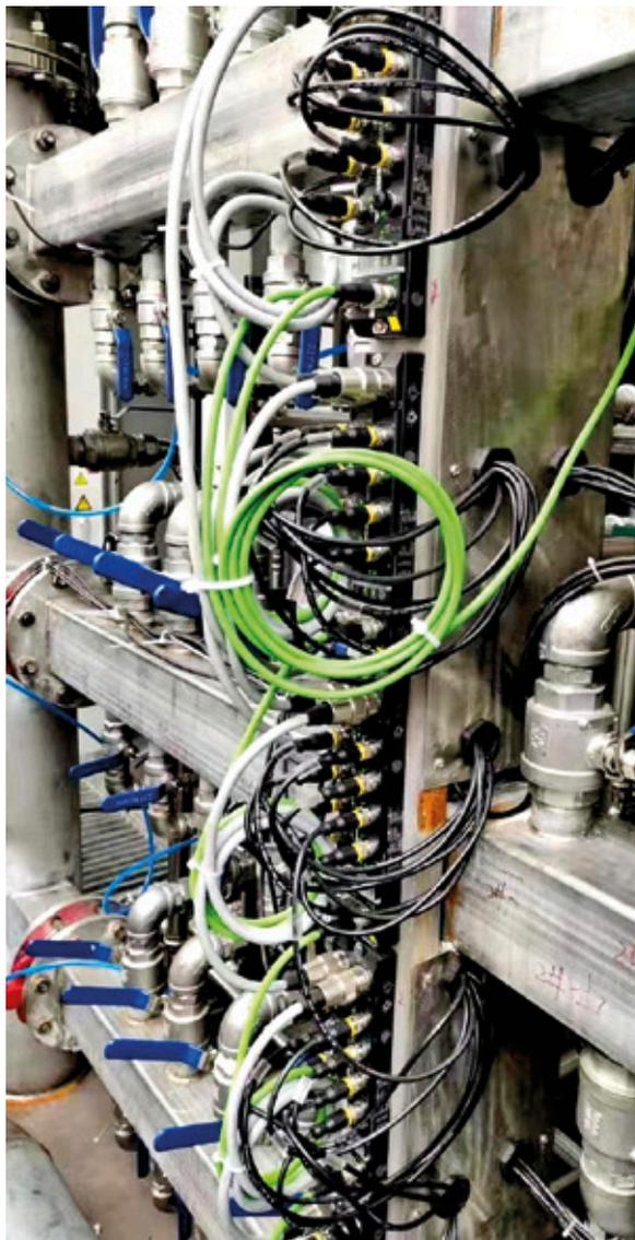
Relevant process data and measured values are transmitted to the controller via Turck's IO-Link master
